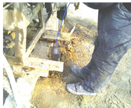
Fig. 9 Field installation of micro-seismic sensor.
