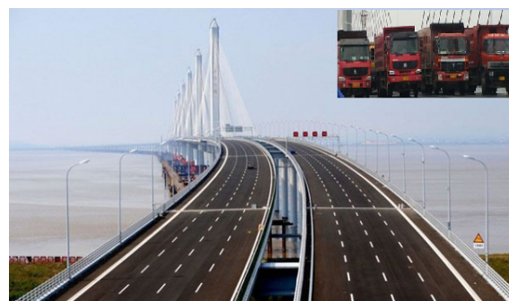
Fig. 7 Overview of a bridge across the river in China.
