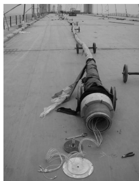
Fig. 3 Smart cable used in real bridge engineering.
