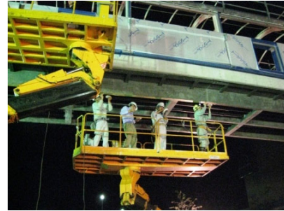
Fig. 13 Optical fiber sensor installation on girder.
