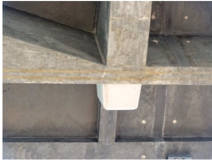
Fig. 16 Mounted five-year-old optical fiber.
