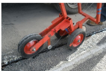
Feeding the strain cable into the slots
