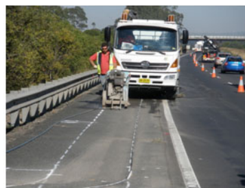
Saw cutting the slots
