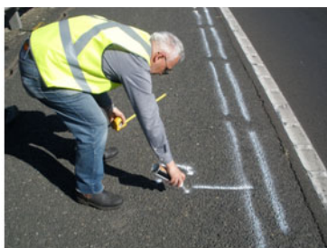
Marking out the site
