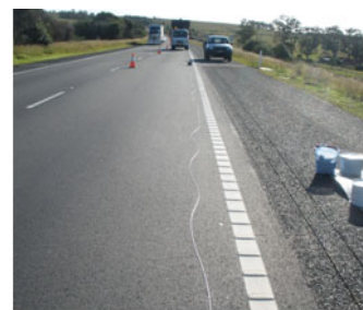
Unspooling the temp cable
