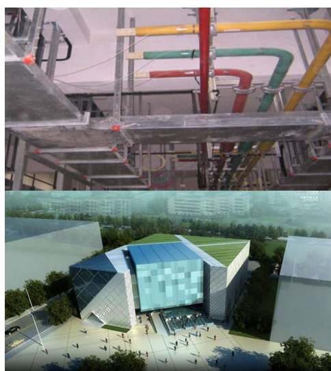
Fig. 16 Setup of the 110-kV ultrahigh voltage Mengzi underground transformer substation of Shanghai World Expo’s fair.
