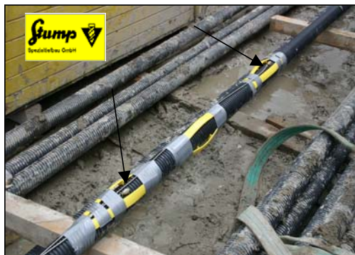
Fig. 21 Prefabricated anchors with fixed pH sensors (arrows).
