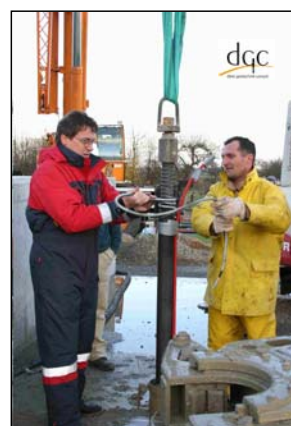
Fig. 10 Introduction of the micro pile into the bore hole.
