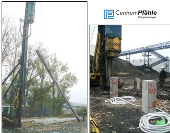
Fig. 5 Precasted sensor-equipped piles before and after driving process.
