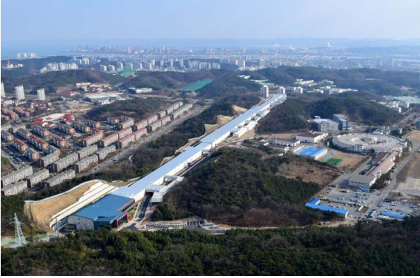
Figure 1. Construction site of PAL-XFEL.
