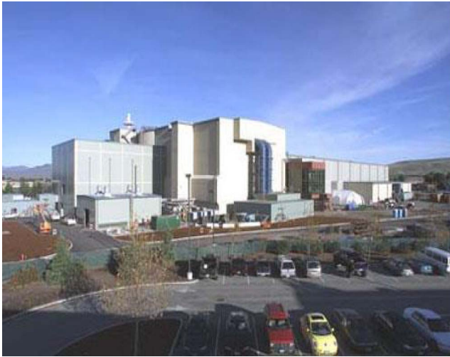
Figure 6. The NIF facility at LLNL, California, USA (picture courtesy of LLNL).
