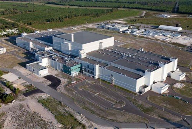
Figure 7. The LMJ facility in Bordeaux, France (picture courtesy of CEA).
