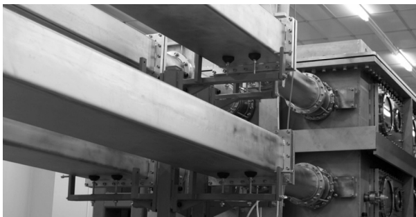
Figure 10. Beams bounded together preventing error accumulation.
