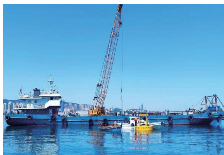
(a) 现场布设 (a) On-site deployment
