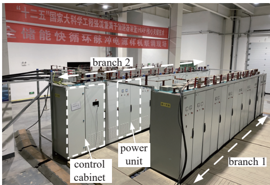
(a) prototype of HIAF-BRing fast cycle full energy storage pulse power supply
