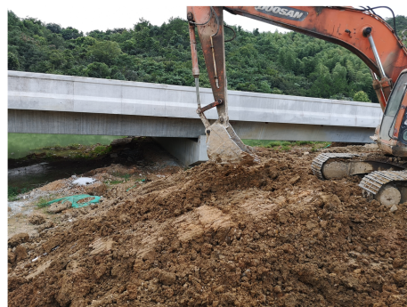
(c) Excavator exerts force on the slope
