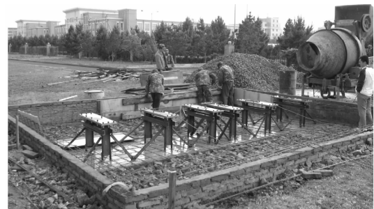
(a) Fix pre-embedded piece of ground base
