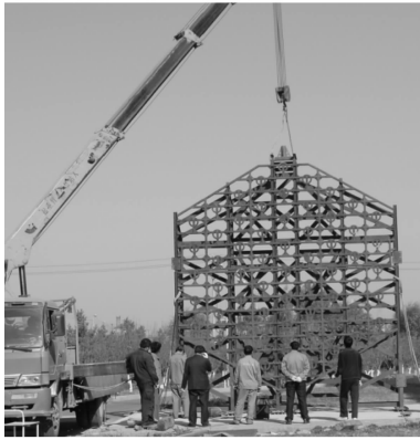
图 5 支撑桁架组装后整体吊装 Fig. 5 Integrated suspending truss after assembly
