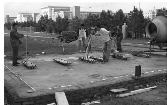
(b) Measure planes error of pre-embedded piece
