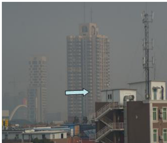
Fig. 3. Photograph of building to fix target and the arrow indicates the position of target.
