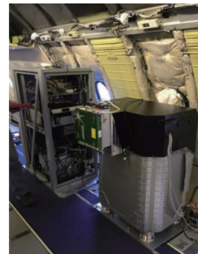
图 5 机上激光终端 [21] Fig. 5 AOC installed in Airbus A310 [21]
